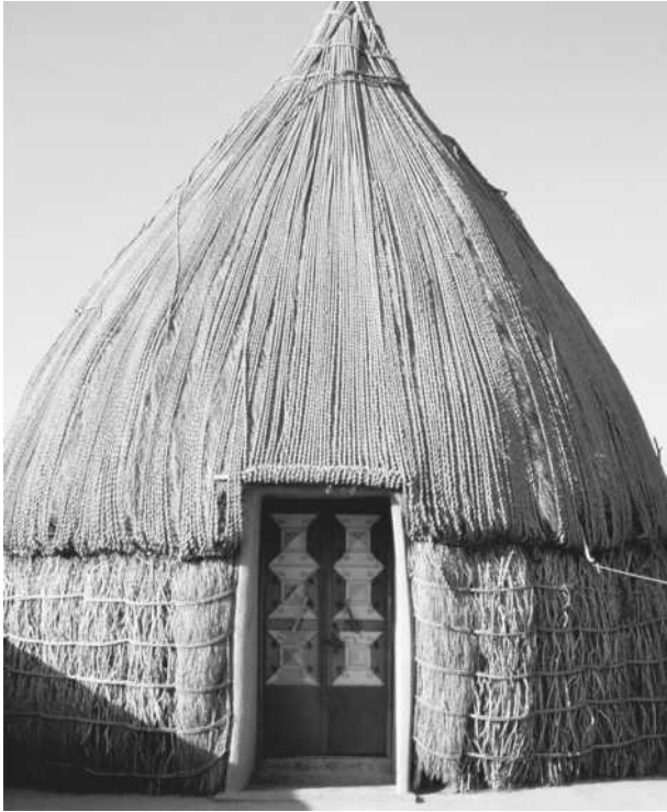
A traditional Yemeni hut in the village of Tihamah uses timber and straw.
